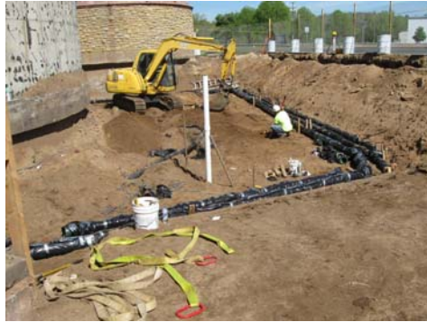
Above, relocation / installation of new air line piping. Below, Supervisory Controls And Data Acquisition (SCADA).
