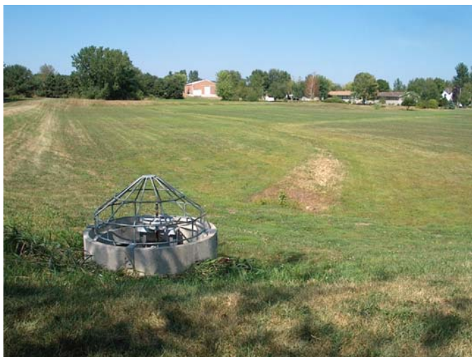
Expanded storm water detention basin doubled the storage capacity.
