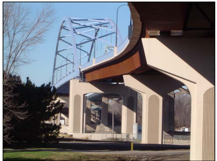
The two previous bridges over the Mississippi River at La Crosse were completed in 1891 and 1939 (shown in top photo). Cedar Corporation designed nine substructure units for the new bridge (shown in bottom photo).
