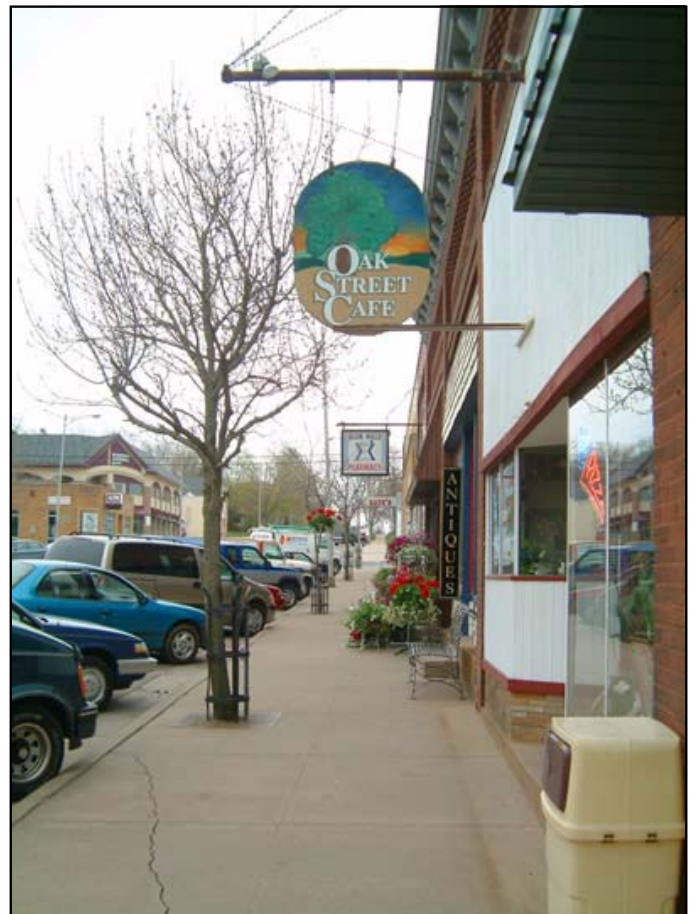
The downtown streetscape will see improvements such as new sidewalks with concrete brick pavers, metal trash receptacles to replace lightweight plastic trash bins, and antique-style benches and street lights.
